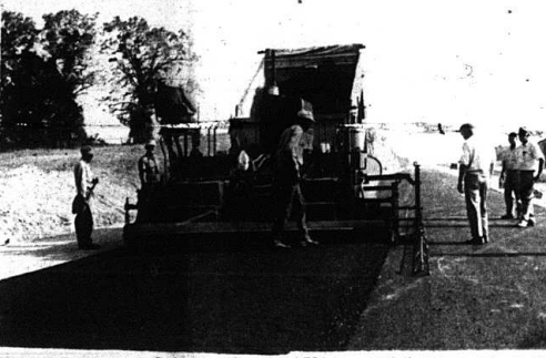
PAVING INTERSTATE - Paving is underway on I-75 between Brindle Ridge and the Renfro Valley Interchange. When paving is completed, the interchange will be open to the Burr Interchange, just south of Mt. Vernon. Allen Co. of Winchester is the paving contractor.
