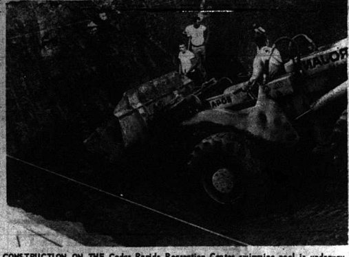
CONSTRUCTION ON THE Cedar Rapids Recreation Center swimming pool is underway. The above photo shows workers removing dirt from where the pool will be located. The bottom photo shows the progress made on the golf course at the No. 5 green.
