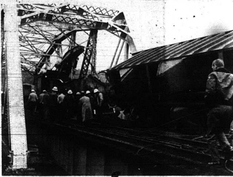
FIFTEEN CAR DERAILMENT-- Sheriff Tip Reppert is shown examining the wreckage of a fifteen L & N freight train car derailment which occurred about 11 p.m. Monday, October 28 just south of Livingston. The cause of the derailment is not known, according to an L & N official. The train, eighty cars long, was loaded with coal heading to Cincinnati from Corbin. There were no injuries from the derailment and there was no estimate of the damage made at press time of the Signal by L & N.
