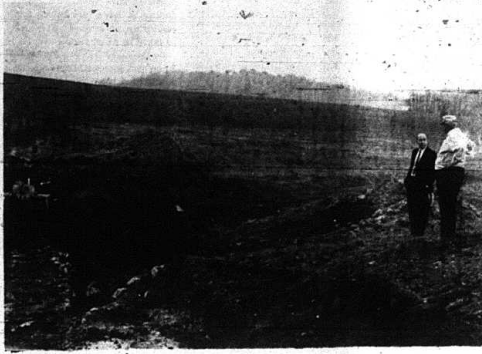
DR. GEORGE GRIFFITH, right, and Bill Bayly of Mt. Vernon watch the progress being made on the dam at Cedar Rapids Recreation Center. The dam will form a small lake and water for the golf course will be piped from it. Work is progressing smoothly on the entire project with the clubhouse almost under roof.
