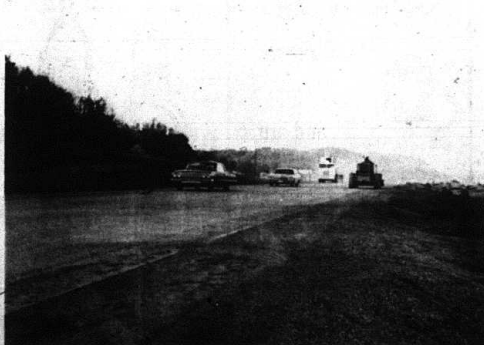
INTERSTATE 75 OPENS -- The southbound lane of I-75 from Conway to Remko Valley was opened to traffic Tuesday morning. In the above photo, construction crews are shown working on the temporary interchange at Conway which they will finish removing in about 10 days. Northbound traffic may go onto I-75 at Burr but will have to get off at Remko and continue on to Beree by old U.S. 25.
