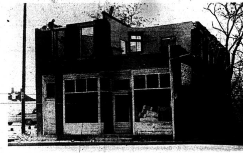
BUILDING BEING RAZED —The two story brick building, located on Richmond Street next to the City Parking Lot, is being torn down. Estil Hodges, local Western Auto store, plans to erect a new building on the site. The building is believed to have been built in 1917 or 18 and Neil Porrett was reportedly the contractor.
