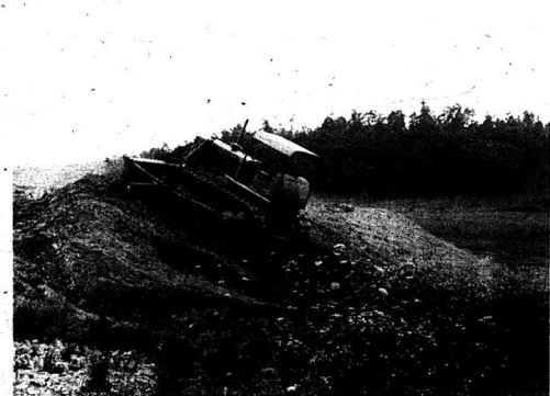
DOCK CONSTRUCTION BEGINS. Work has begun at the site of the City Boat Dock on Lake Linville. Pictured above is Guy C. Martin of Mt. Vernon who is doing the preliminary bulldozer work on the dock.
