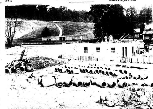
NEARS COMPLETION. Construction of the new water treatment plant at Reno Valley pictured above is about three-fourths complete; however, Lake Linville must rise about ten feet more before any water can reach the lower intake on the intake stand shown in the lower photo. How long it will take the lake to reach this level naturally depends on the amount of rainfall we get. The lake has risen considerably since the valve was closed about three weeks ago.
