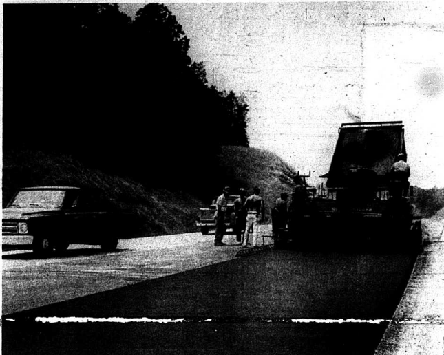
PAVING INTERSTATE —Simultaneous surfacing of Interstate-75 between the Burr Interchange and Rockcastle River is progressing rapidly. The main traffic lanes should be completed next week. The next section of the
