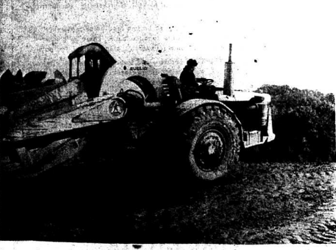
QUA! DUCK PROGRESS -- Progress is being made on the City of Mt. Vernon's Boat Dock at Lake Linville. Pictured above is the concrete pump already paired. In the bottom photo, a piece of heavy equipment, operated by Guy C. Martin, dumps a load of dirt.
