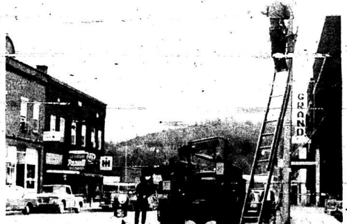
PUTTING THE LIGHTS UP— Kentucky Utilities workers were busy Tuesday afternoon stringing the new Christmas lights across Main Street in Mt. Vernon. The lights were purchased by the Mt. Vernon Businessmen's Association and there will be a formal lighting next Friday night, the 28th.
