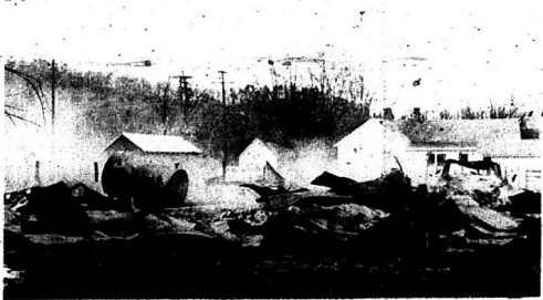
Fire completely leveled the above barn and destroyed all contents shortly after midnight Monday night. The barn, located across from Sowder Nursing Home in Brodhead, was approximately twenty years old.
