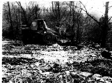
CLEANING IT UP, AGAIN —This scene was repeated throughout the county last week in an effort by the State Highway Department to get rid of some of the piles of trash dumped illegally on the side of roads by county residents. The photo was taken on the property of Paul Baker near the intersection of U.S. 25 and Chestnut Ridge Road and is the same site as the photo run in last week's Signal. The State brought in tons of dirt, buried the trash and then "walked" it down.
