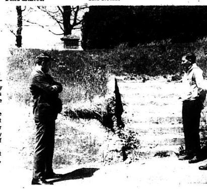
Three members of the Rockcastle County Jaycees look over a portion of the wall around Elmwood Cemetery in Mt. Vernon which is crumbling. The wall is in bad disrepair all over and the Jaycees have begun a drive for funds to repair the wall. Shown in the above photo from left: William D. Gregory, David Henderson, and Buddy Cox.
