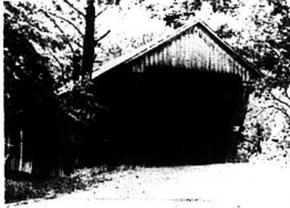
TYGART'S CREEK BRIDGE ... in Greenup County
