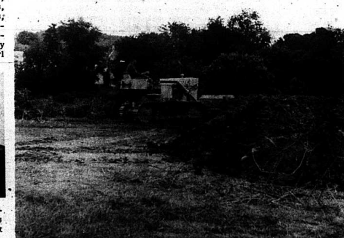
Remember when the star quarterback crossed the 50-yard line on Mt. Vernon's football field and had to back up 20 yards? Well, this event might not occur anymore if plans as according to schedule. Jimmy Cromer, of Mt. Vernon, bulldozer operator, is shown filling in one end of the field and plans are to complete it to a regulation 100-yard length in time for the football season.
