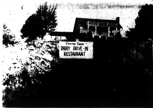
The above construction is going on a U.S. 25 just north of Mt. Vernon near the Renfro Valley Interchange of I-75. Upon completion, it will be a drive-in restaurant. The site is owned by William K. and Mary O. Cummins. TOM DUNCAN'S
