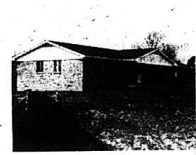
Mr. and Mrs. Rustin's home, with electric heat installed, was built in 1969.
