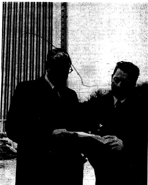
PLAZA TOWER—Finance Commissioner Albert Christen, left, and Al Hubbard, Christen's assistant, have been named to prepare the 28-story Capital Plaza tower for occupancy by some 1500 state employes. Workers are now preparing to roof the tower, and the state may begin moving into the new facility as early as December of this year. (Jim Toole Photo)
