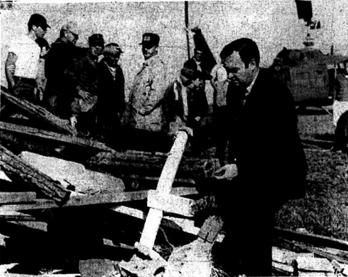
EXAMINES DAMAGE —Governor Louie B. Nunn examines a wrecked building in Adams County near Columbia. The shattered structure was one of hundreds of homes and other buildings destroyed when tornadoes struck six south central Kentucky counties Tuesday night taking at least ten lives. (Ronnie Manns photo)
