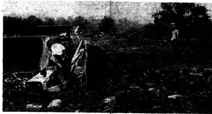
Workers for the McGregor and Neal Construction Co. of Lexington are shown beginning construction on the new sewer disposal plant for the City of Brodhead. The plant will be located between Soward Nursing Home and the old swinging bridge on land formerly known as "Robbins Bottom."
