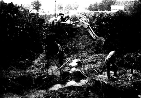
Workers for the J.M. West Construction Co. of Cookeville, Tennessee, contractors for the water line project in Broadhead, are shown as they cross Negro Creek with the line near Farmers Feed Mill. This part of the water and sewer project, also scheduled for completion by June 1, 1972, along with construction of the sewer lines and sewer plant are being financed by a loan and grant to the City of Broadhead from the federal government.
