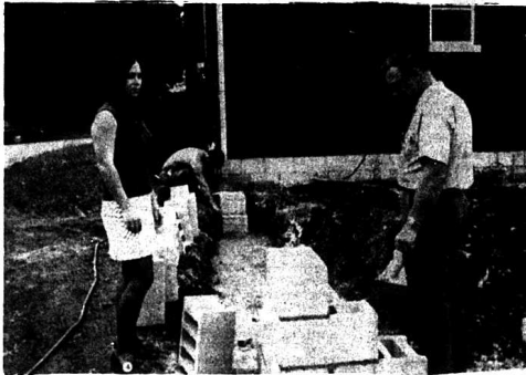
Mrs. Jerry Hanel, PCA secretary, and Roy Brown, PCA manager, look over the masonry work in progress on the addition to the present Cumberland Production Credit Association building on Main Street in Mt. Vernon. According to Mr. Brown, the new addition will be 20' x 32' and will be used as an Agri-Business Conference Room. The building should be completed sometime this fall. Virgil Abney, also shown in the above photo, and James Krenthel Abney are doing the masonry work on the building and the contractors are W.E. Procter and son.
