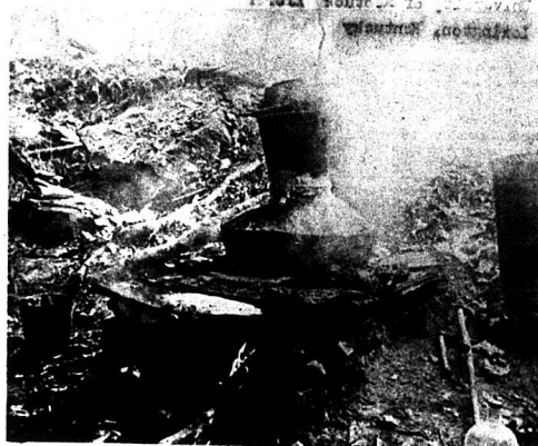
MOONSHINE STILL IN OPERATION--This photograph of a moonshine still in operation, showing the cooker while the fire is under it, is one of the more than 650 pictures featured in "Kentucky: A Pictorial History," to be published this month by the University Press of Kentucky.
