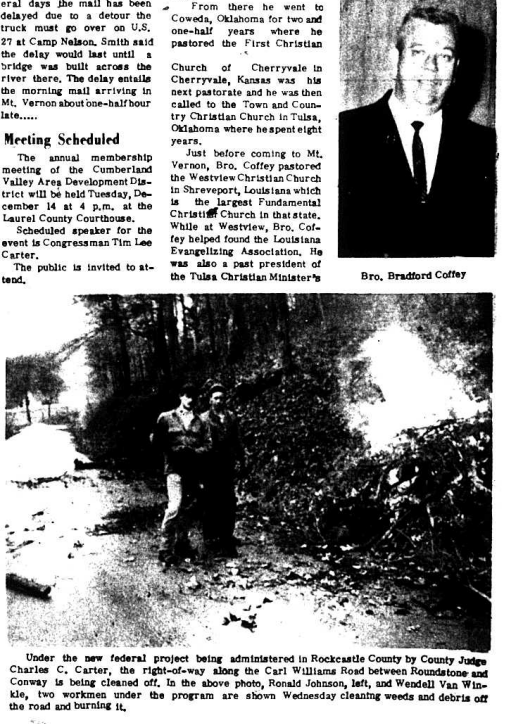
Under the new federal project being administered in Rockcastle County by County Judge Charles C. Carter, the right-of-way along the Carl Williams Road between Roundstone and Conway is being cleared off. In the above photo, Ronald Johnson, left, and Wendell Van Winkle, two workmen under the program are shown Wednesday cleaning weeds and debris off the road and burning it.
