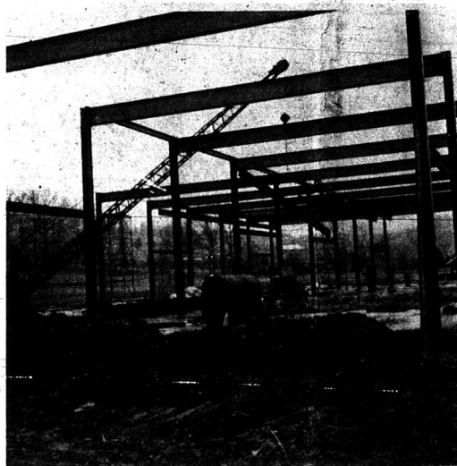
Billy P. Cass of Broadhead is the contractor for the new building presently under construction by the Clow Corp. on U.S. 150 between Mt. Vernon and Broadhead. The new facility will contain 16,000 square feet and will double the
