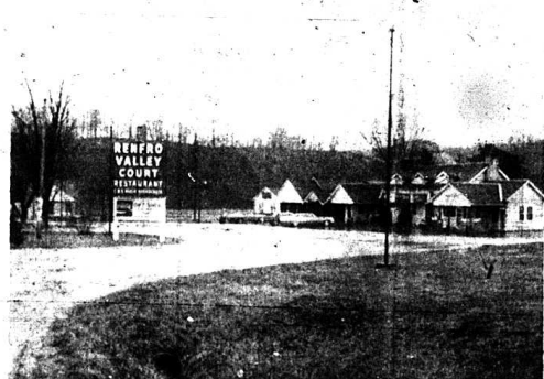
Saturday, February 20, the largest private construction contract that it is believed has ever been let in Rockcastle County was completed at the Bank of Mt. Vernon between Alpha Smith and Renovo Valley and Bromwell-Kesterson Construction Co. of Knoxville, Tennessee after 18 months of negotiations. The contract, for more than one-quarter of a million dollars, calls for the construction of a forty-unit double-deck motel, a swimming pool and sewer and water lines on the property. The motel is scheduled to be in operation by June 15 of this year. The motel is located on the site of the former Renovo Valley Lodge and Restaurant behind the Texaco Service Station. When the project is completed, Mr. Smith's facilities in Renovo Valley will consist of the forty-unit motel, thirteen cabin units, the pool and a dining room in the Lodge which seats over 200 people. The above photo shows the present lodge. The new motel will be located just adjacent to it. A portion of the hill in the background of the picture will be cleared for large signs that will be visible from I-75.
