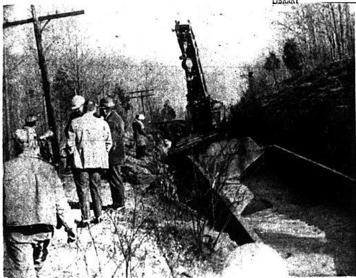
L & N Wreck Crews were still trying to get the tracks cleared Friday from a 33-car wreck which occurred last Tuesday just south of Mt. Vernon. Crews worked from both ends of the pile-up removing wrecked cars and laying new track. Cars were unloaded and pushed off to the side. Monday of this week was the first day that a train could be routed through here.
