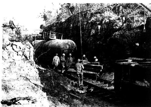
L & N Wreck Crews were still trying to get the tracks cleared Friday from a 33-car wreck which occurred last Tuesday just south of Mt. Vernon. Crews worked from both ends of the pile-up removing wrecked cars and laying new track. Cars were unloaded and pushed off to the side. Monday of this week was the first day that a train could be routed through here.
