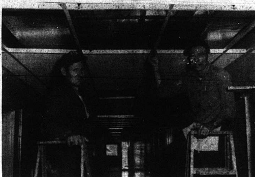
AIR CONDITIONING FOR HOSPITAL - Luster Bullock, left, and Ed Burke, workmen for the county's EEA program are shown installing some of the air conditioning ductwork in the Rockcastle County Hospital. To date, the hospital has paid for and is installing four units, which cost approximately $5,000 besides the ductwork. It takes five units to completely air-condition the hospital but funds are not available to purchase the fifth unit plus some other needed supplies, which would run the total needed for completing the project up to approximately $5,500. The ceiling being installed over the ductwork is 3/4" fire rated ceiling made of non-combustible material. The men are installing the system under the supervision of Brock-McVey Co. and the four units are expected to be ready for the hot weather.
