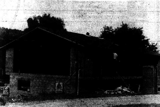
An Office Building and Apartment Complex, being constructed by Dr. Orson Arvin, adjacent to the Rockcastle County Hospital, is expected to be completed sometime in the fall. Dr. Arvin's office will be upstairs with two apartments underneath. Burllyn G. Calder of Corbin is the contractor for the 30 x 58 building.
