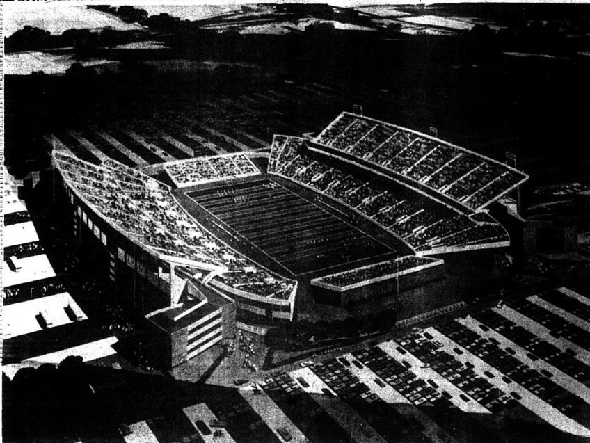
The University of Kentucky's new Commonwealth Football Stadium (Capacity 58,000) which is expected to be completed in September of 1973.
