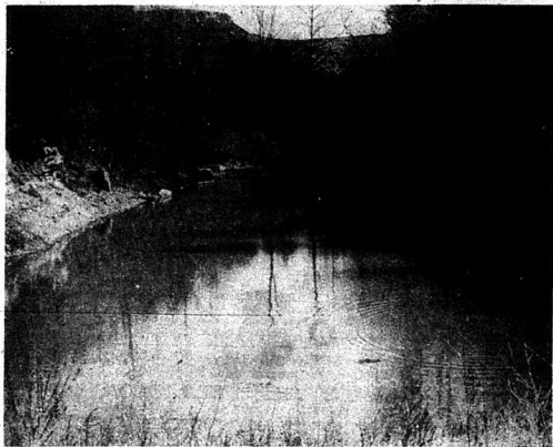
SILT DAMS —Hundreds of silt dams on strip mining operations throughout Kentucky prevent dirt from running into nearby streams. According to Thomas O. Harris, commissioner of the Kentucky Department for Natural Resources and Environmental Protection, regulations passed by the Division of Reclamation in the last several years have reduced the causes of erosion and silt dams have caused most of the run-off to be retained on the mine site.
