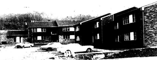
ROCKCASTLE VILLA, a 48-unit low-income housing project on the Old Brodhead Road, is scheduled for completion within the next month. The FHA financed project will include one, two and three-bedroom units. Applications for renting the units, a portion of which have been set aside for the elderly, may be made daily, Monday through Friday, from 9 a.m. to 1 p.m. at the office located in the project. Tommy Parsons is serving as Director of the Project and may be reached by calling 256-4822.
