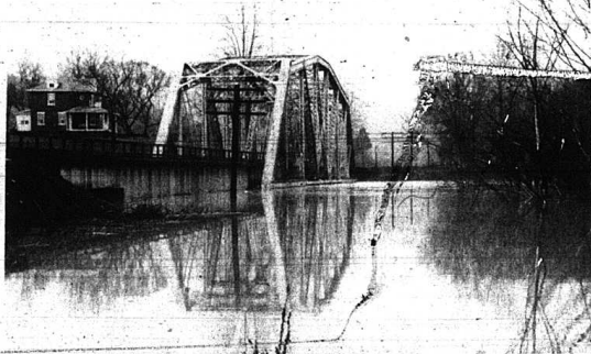
HEAVY RAINS caused problems all over Rockcastle County last Thursday morning and especially at Livingston where the above photo was taken. The scene is the L & N Railroad bridge there about noon Friday at which time the water had dropped about six inches from its peak stage. Some residents of the area claimed that the water was as high as they had ever seen it while other residents said they had never seen the river higher. Others told of seeing, several years ago, three engines sitting on the bridge in order to keep it from washing away. However, it is believed that since that time, the bridge has been raised.
