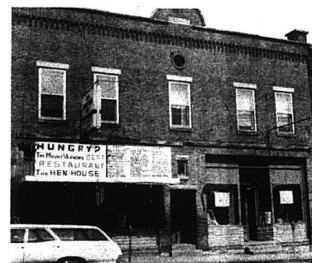
Good business building located on Main Street in Mt. Vernon, KY. This building is completely rented bringing in a good rental income. Ideal for quick sale.
