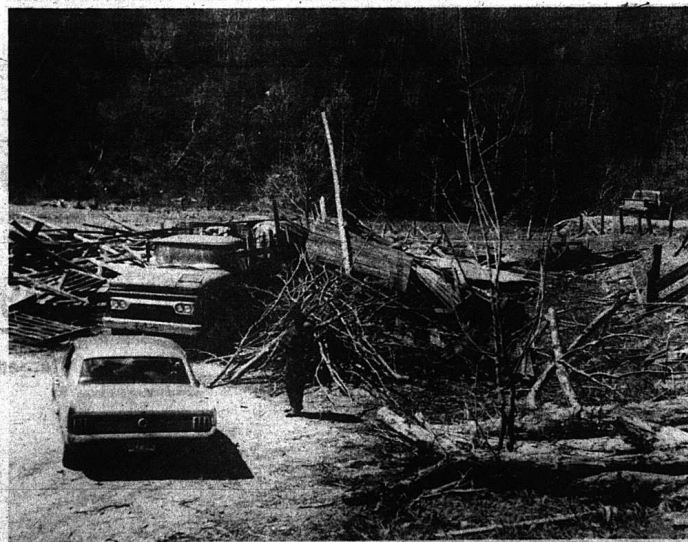
The remains of the barn, located at the home of J. W. Gilliam at Lamero, are shown in the above photo. Mr. Gilliam's home was also damaged, and a chicken house and chickens and a hog house
