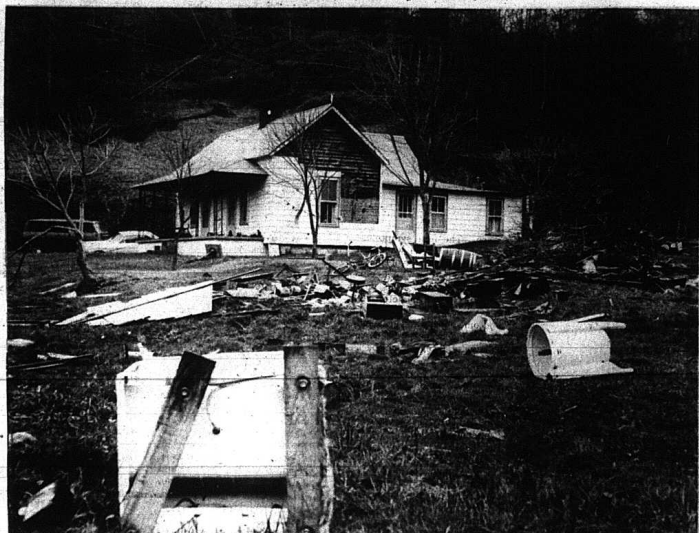
The Morris Robinson residence on Trace Branch Road also suffered heavy damage during Wednesday night's tornado. Besides heavy damage to their home, their barn and three outbuildings were destroyed. One of the outbuildings housed their
