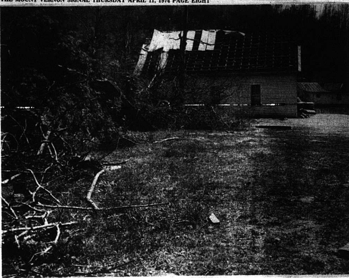
Mr. and Mrs. Ed Coburn of Trace Branch took refuge in the basement of the Pleasant Run Church only to be injured by flying debris when the church was struck and destroyed by the tornado.
