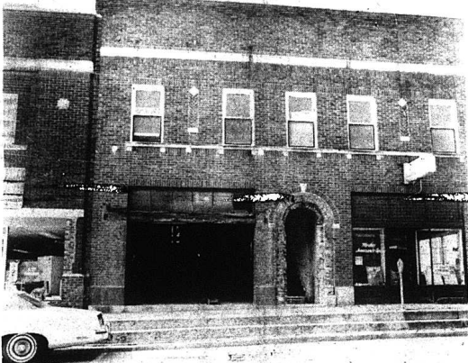
ANOTHER TOWN LANDMARK is leaving the scene. A renovation project on the old Vernon Theatre Building, by its present owner Clarence Carter, will finally close the doors on what was, until the last few years, the entertainment center for Rockcastle Countians. The building was originally constructed in 1927 by Milton J. Miller and opened with a silent movie entitled "Men of Steel" starring Milton Sills. The movie at that time ran with the only sound coming from a three-piece orchestra - Mr. and Mrs. Bragg Thompson and son, Robert Huffman. About 1933, along came sound and the Vernon installed the "novel" device. The Vernon Theatre was operated by the Miller family until 1962, except for a short time during the 1930's. According to Mr. Carter, the building will be renovated with apartments upstairs and the lower floor rented out to a business.
