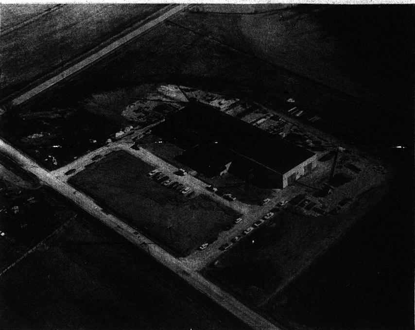
Aerial view of 44,000 square foot steel fabricating facility near Broodhead that has been leased by Braden Steel Corporation for the manufacture of silencing systems for the power generating industry.
