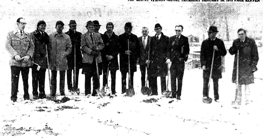
The Building Committee and congregation of the Wildie Christian Church braved cold temperatures and falling snow to hold a ground-breaking ceremony Sunday at Wildie. The church plans to begin construction of their new 7,000 square foot sanctuary right away. Members of the building committee shown in the above
