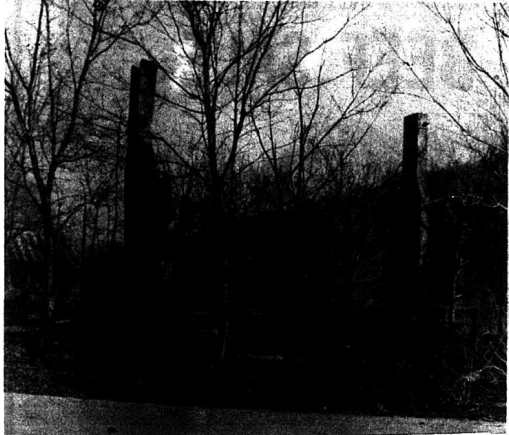
Vandalism was apparently the cause of a fire which completely destroyed an unoccupied two-story frame dwelling on the farm of Matt Coffey, 7 miles east of Mt. Vernon. The house was the home of the late Johnny Coffey.
