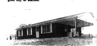
COUNTRY LIVING - Modern home - 3 bedrooms - wall to wall carpet - ceramic bath - electric heat - plus much more - Hard to believe - All for only $21,500.
