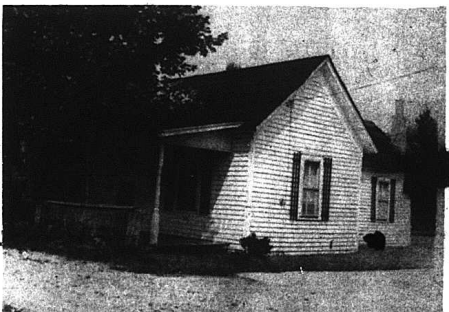
House #2 - Has 3 bedrooms, living room, kitchen and bath. It also has storm doors and windows and city water and sewer.
