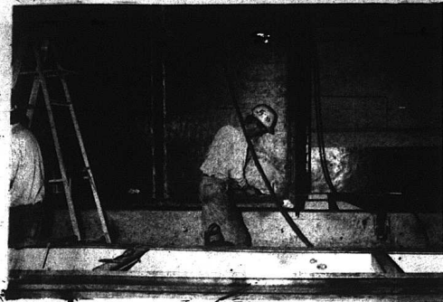
Frankie Jones is shown welding wells on an inlet silencer duct.
