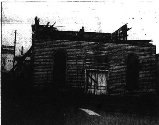
One of the oldest buildings in Mt. Vernon is coming down. The Henderson Family has decided to demolish the building, occupied for many years as the office of the Mt. Vernon Signal, to improve the property and Roman McFerron of Mt. Vernon is contractor for the project. The building, which is approximately 115 years old, was originally occupied as a Christian and Baptist Church simultaneously and also, at one time, the Masonic Lodge occupied the upstairs.
