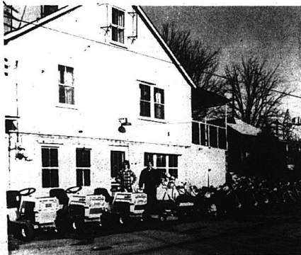
NEW BUSINESS —Roger Nichols and Orville D. Gregory are shown in front of their Cycle Shop which they recently opened in the Percival building on Fairground Hill in Mt. Vernon. In addition to selling cycles, they are carrying a line of riding, self-propelled and push mowers and will also service and repair cycles, chainsaws, lawn mowers, golf carts, etc. (See ad elsewhere in the Signal.)
