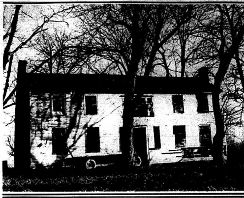
The Mordica Lincoln home in Washington County. The house, last lived in 1953, was built by an uncle of Abraham Lincoln in 1797. The original log cabin structure was covered with the current weather boarding by other tenants in 1815. The Kentucky Department of Parks and the Washington County Historical Society have entered into an agreement to restore and maintain the home as a part of Lincoln Homestead State Park.
