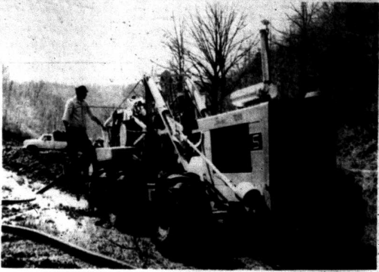
This giant-sized trenching machine, which is owned by John Price and Sons, of Liberty has recently been used to complete the installation of almost five miles of plastic tile to drain wet land in
