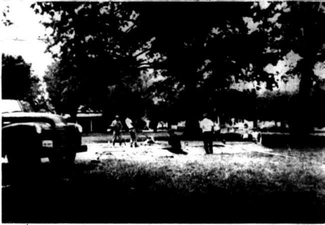
Construction has begun on a new city park for Brodhead located near the elementary school. Shown in the photo working on the foundation for a picnic shelter are, left to right: James Dooley, Frank Glovak, Lagson Whit, Bill Gentry and John Glovak. The park is funded by a federal grant of $2,200 and city matching funds. In addition to the picnic shelter, there will be a
