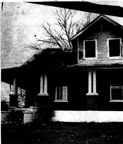
This photo shows the exterior of the house where the fire burned through the roof of the Buswell home in Brodhead early Saturday morning. The home, occupied by Mr. and Mrs. Billy A. Buswell, his three children and two elderly ladies being nursed by Mrs. Buswell was completely destroyed by the fire which began in the flue of a downstairs fireplace. The Buswell family had been remodeling the home for some time and it was almost completed at the time of the fire.
