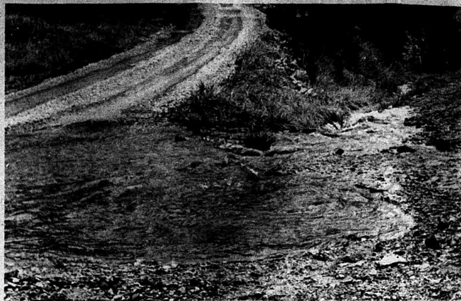
William D. Gregory, local attorney, and water lines just don't seem to get along. The above photo shows Mr. Gregory's driveway at his home on U.S. 25 which was flooded due to a broken water main last Friday. The photo at right shows
