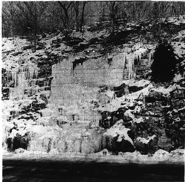
One of the most spectacular winter scenes in Rockcastle County is the cascading icicles formed in the cut on Burr Hill. The water comes from tiny underground streams which find an outlet in the limestone cliffs made when the roadway was built. Thus far, a low temperature of three below zero has been recorded this year and, on the 11th day of January last year, the low was also
