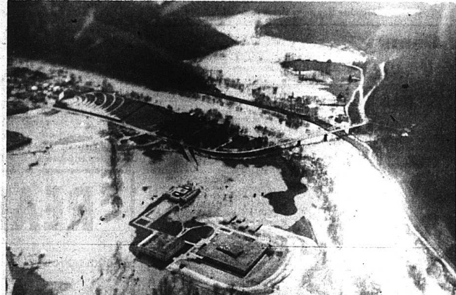
The Levisa Fork Overruns Its Banks filling the valleys and lapping buildings in Prestonsburg. Such scenes are common in many parts of Eastern Kentucky where flooding started earlier last week.
